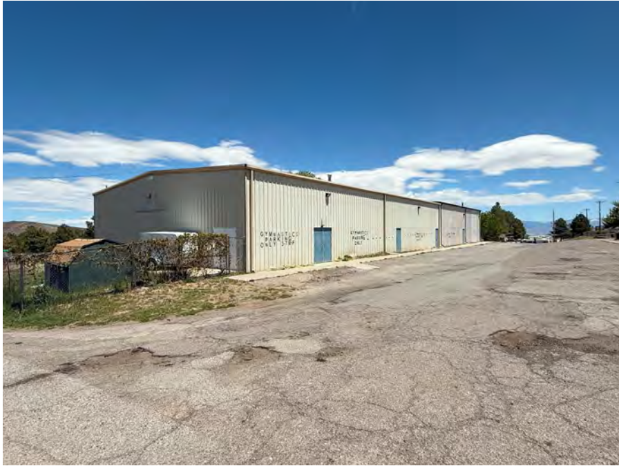
Front view of the subject property looking northeast
