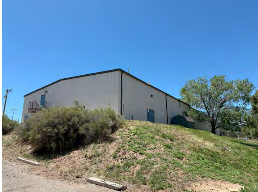
Rear view of the subject building looking southwest
