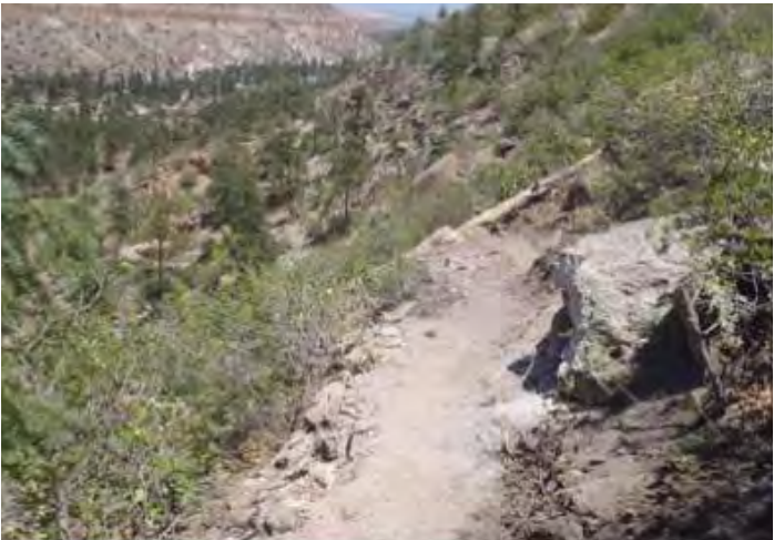
Monitor condition of switchbacks throughout the trail.
