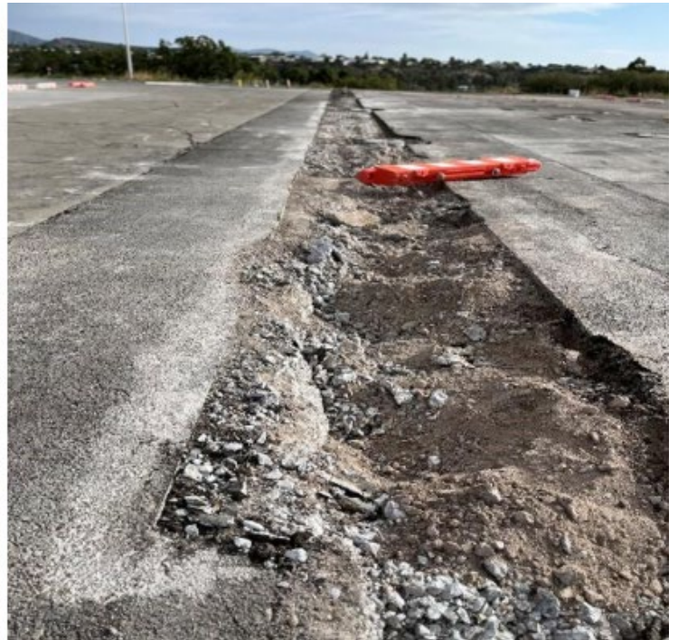
Los Alamos County Airport T-Hanger's Project: Concrete Removal at New Trench Drain Column's Location and Concrete Piers for Steel.
