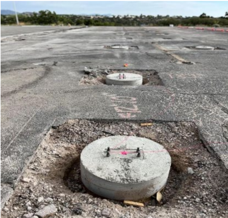
Los Alamos County Airport T-Hanger's Project: Concrete Removal at New Trench Drain Column's Location and Concrete Piers for Steel.
