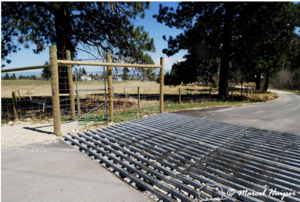
Figure 33. Wildlife guard at an access road to US Hwy 93S, near Victor, Montana, USA. This type of wildlife guard is less suited for pedestrians and cyclists.
