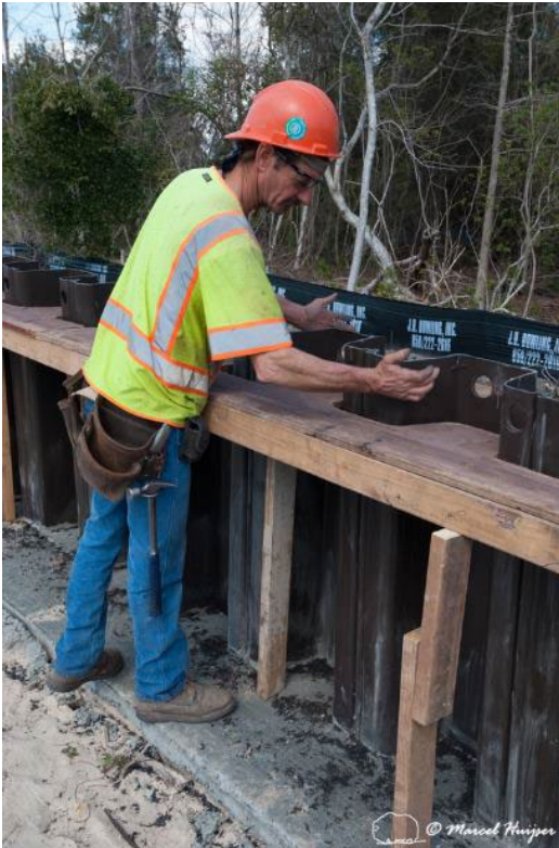
Figure 65. Barrier wall for turtles, alligators, snakes and amphibians, Lake Jackson Ecopassage, Tallahassee, Florida, USA. The barrier wall was under construction when the image was made.
