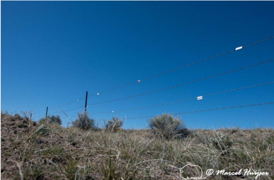
Figure 60. Fence markers (white vinyl strips with or without reflective tape) to increase fence visibility and reduce sage grouse strikes, Montana, USA.
