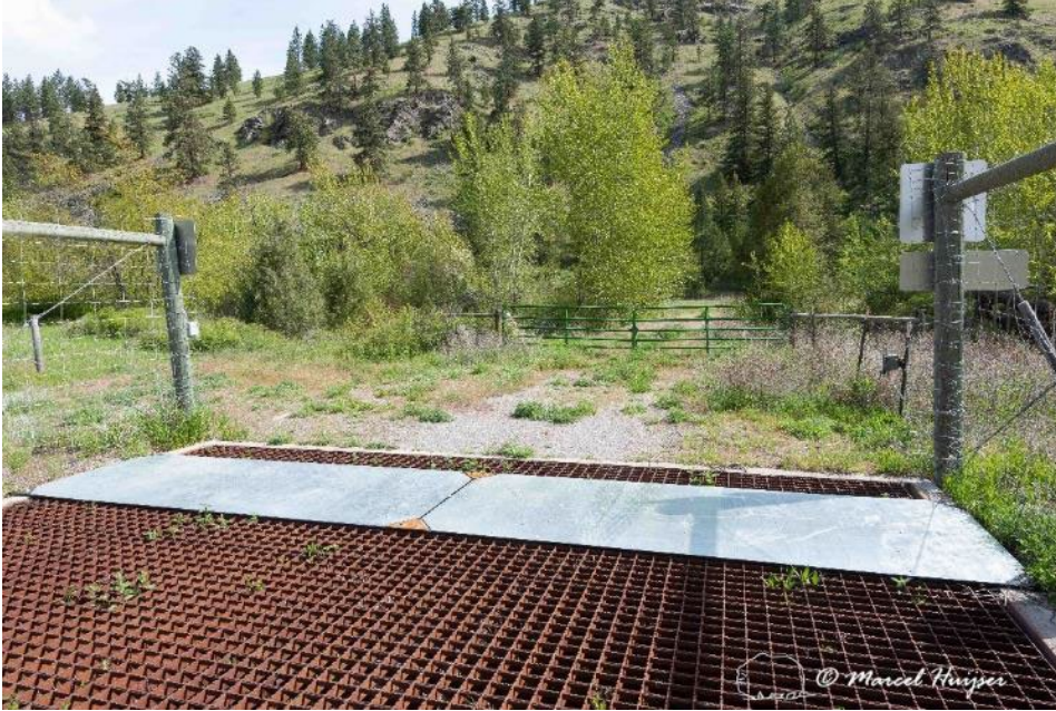
Figure 34. Electrified barrier, designed for low traffic volume and low traffic speed, on top of a wildlife guard at an access road to US Hwy 93S, near Ravalli, Montana, USA.
