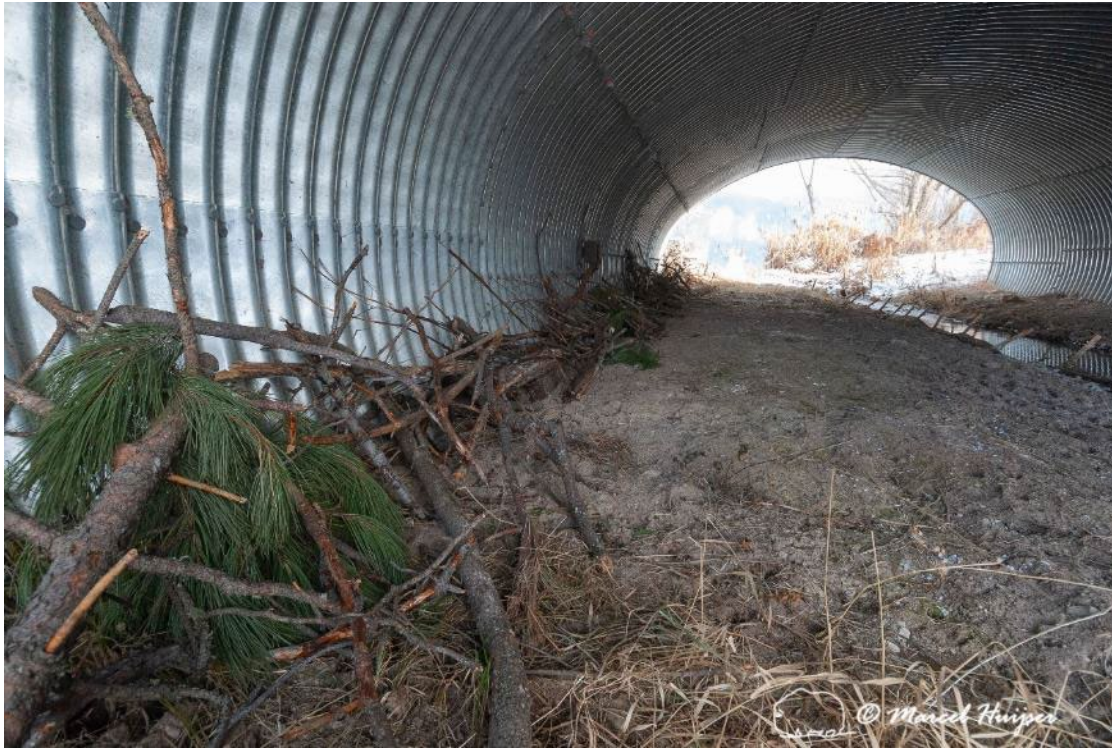
Figure 85. Wildlife underpass with branches along the side for cover for small mammals, Montana, USA.
