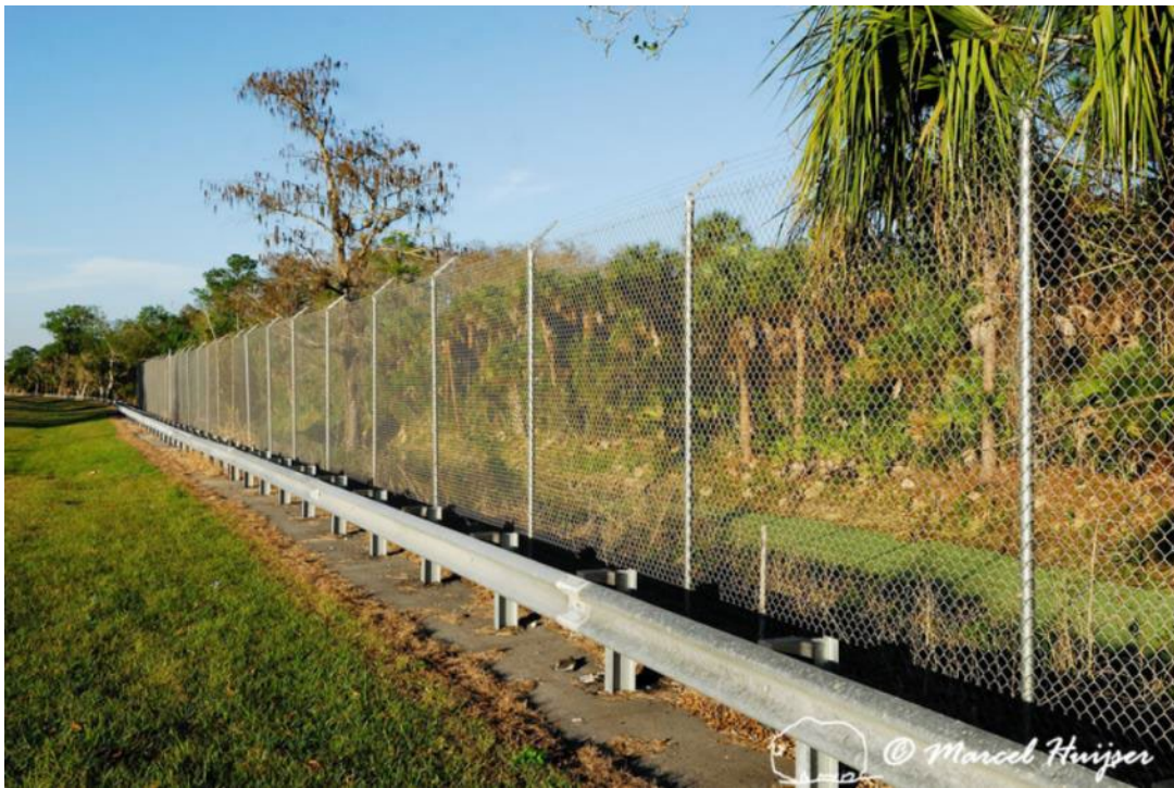
Figure 8. Fence for Florida panther ( Puma concolor coryi ), 10 ft tall, metal posts, chain-link fence material, and overhang, SR 29, Florida, USA).
