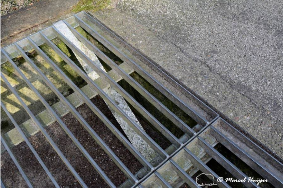
Figure 105. Escape ramp for small animals from pit under wildlife guard National Park Hoge Veluwe, The Netherlands.
