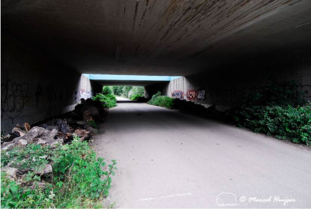
Figure 99. An existing underpass for a low volume road under a 4-lane A27 motorway, near Hilversum, The Netherlands. The structure was made more suitable for small animal species by placing rows of root wads along the sides.
