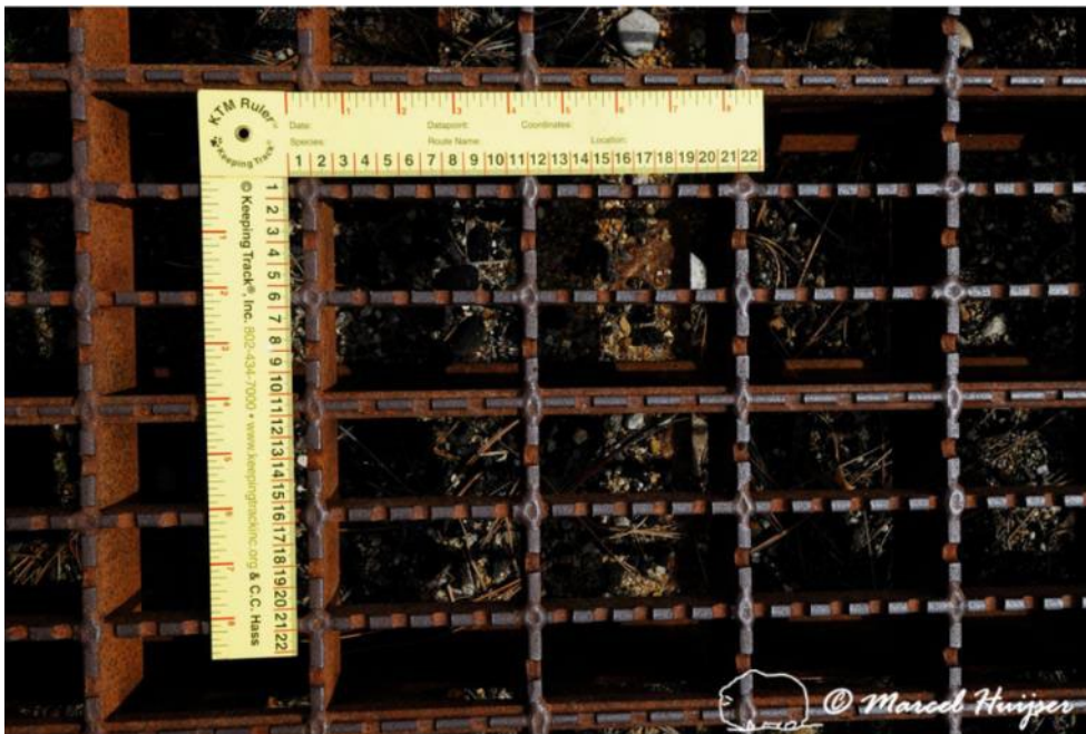
Figure 39. Detail of the modified bridge grate material used for wildlife guards installed at access roads along US Hwy 93, near Ravalli, Montana, USA. This material is more suitable for pedestrians and cyclists compared to the bars of a traditional wildlife guard or cattle guard.
