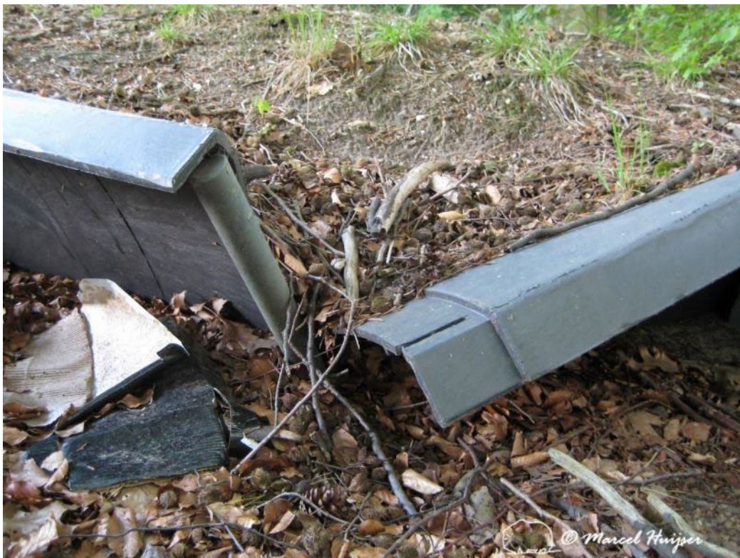
Figure 109. A barrier wall for common toads ( Bufo bufo ) has collapsed, The Netherlands.
