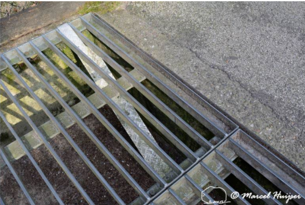
Figure 37. For wildlife guards that have a fully enclosed pit with contiguous walls sometimes wooden planks or metal strips are attached, potentially allowing small animal species to climb out of the pit.
