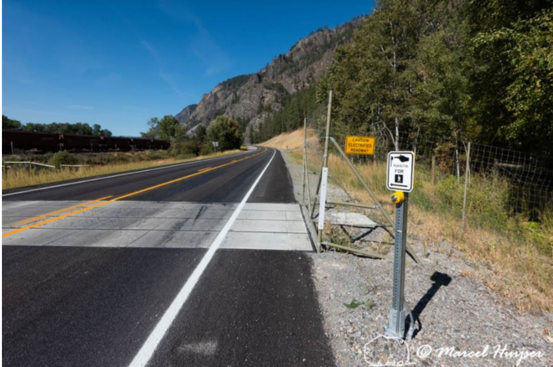
Figure 31. Electrified barrier embedded in travel lanes to keep large mammals, including bighorn sheep, out of fenced road corridor, MT Hwy 200, Thompson Falls, Montana, USA.
