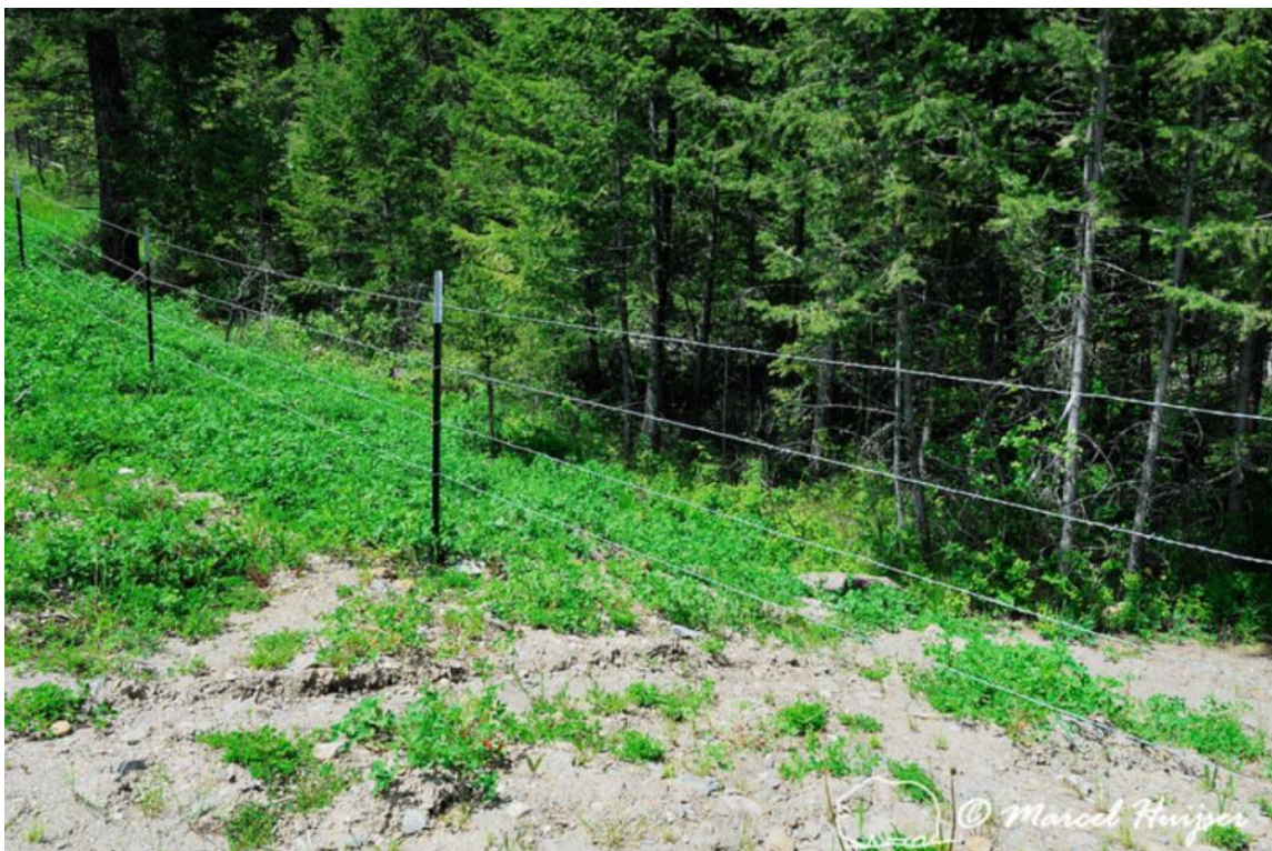
Figure 59. Wildlife friendly livestock fence with smooth top and bottom wires, Montana, USA.
