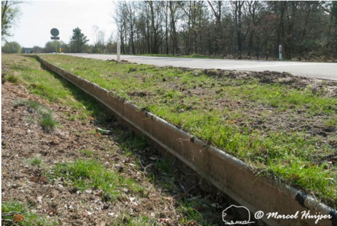
Figure 62. A “barrier wall” (polymer concrete) for common toads ( Bufo bufo ), integrated into roadbed, Deelenseweg, between Hoenderloo and Arnhem, Gelderland, The Netherlands.
