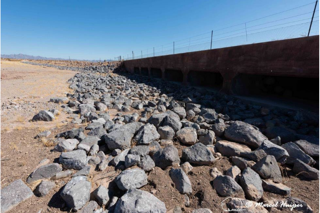
Figure 108. Riprap in front of culverts to reduce erosion, but the boulder are a barrier to Mojave desert tortoise ( Gopherus agassizii ), I-11, near Boulder City, Nevada, USA.
