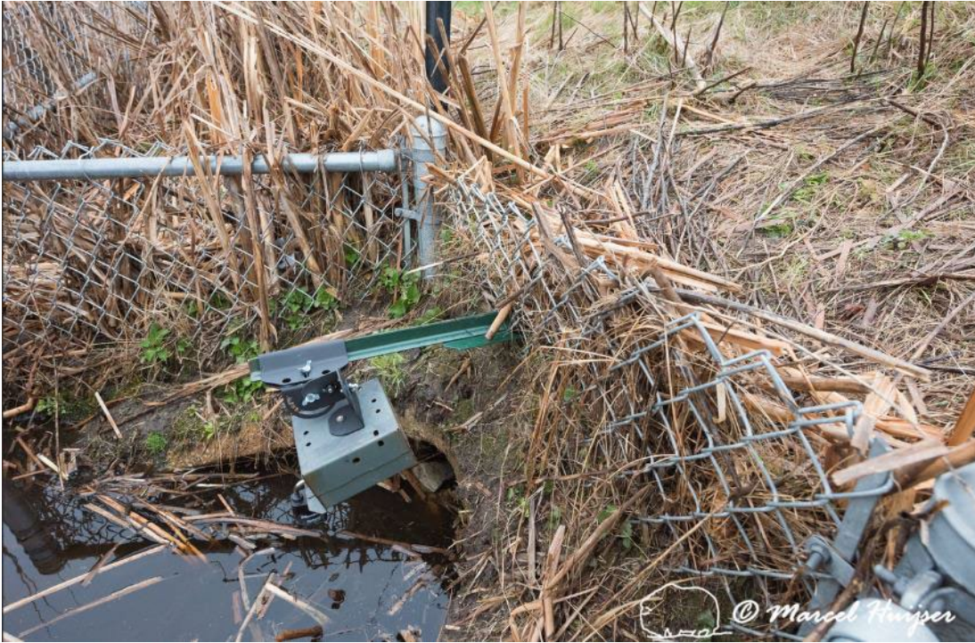
Figure 98. Turtle fence tied into an existing culvert for hydrology, US Hwy 83, Valentine National Wildlife Refuge, Nebraska. The camera monitors potential turtle crossings at the culvert.
