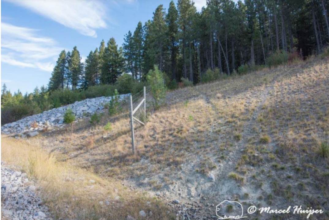
Figure 26. Wildlife trail at a fence-end, US Hwy 95, Bonners Ferry, Idaho, USA. This is an indication that there is a concentration of wildlife crossings at the fence-end (a "fence-end run"), potentially resulting in a concentration of collisions at or near the fence-end, just inside or just outside the fenced road section.
