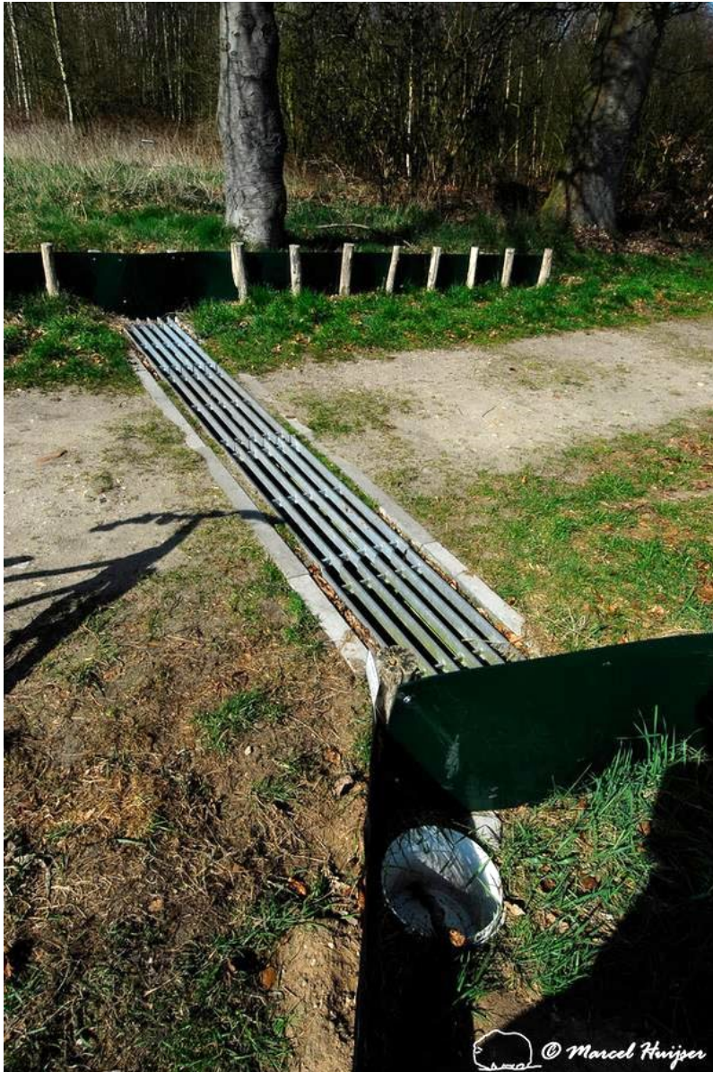
Figure 75. ABS plastic sheets to keep common toads off the highway (highway is to the left of the image), and an amphibian tunnel under an access road. Amphibians that approach the access road would fall in between the bars. Amphibians that travel along the barrier on the other side of the access road until they encounter a tunnel that allows them to cross to the other side of the highway.
