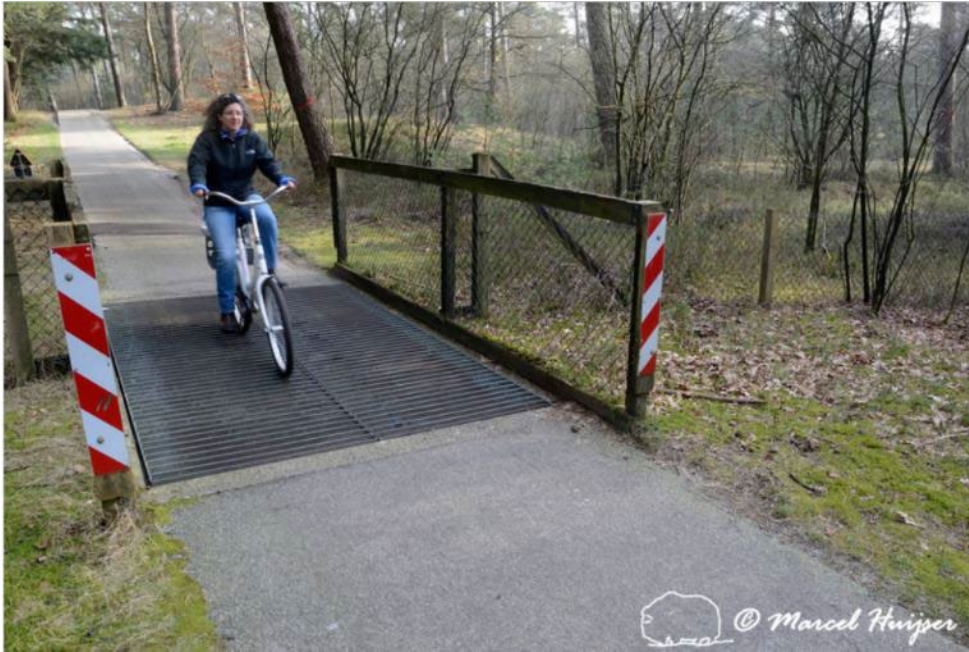
Figure 38. Bicyclist on wildlife guard for wild boar ( Sus scrofa ) and moeflon ( Ovis orientalis ) at a bicycle path, National Park Hoge Veluwe, The Netherlands. This wildlife guard has an escape ramp for small animals that fall into the pit under the metal grate.
