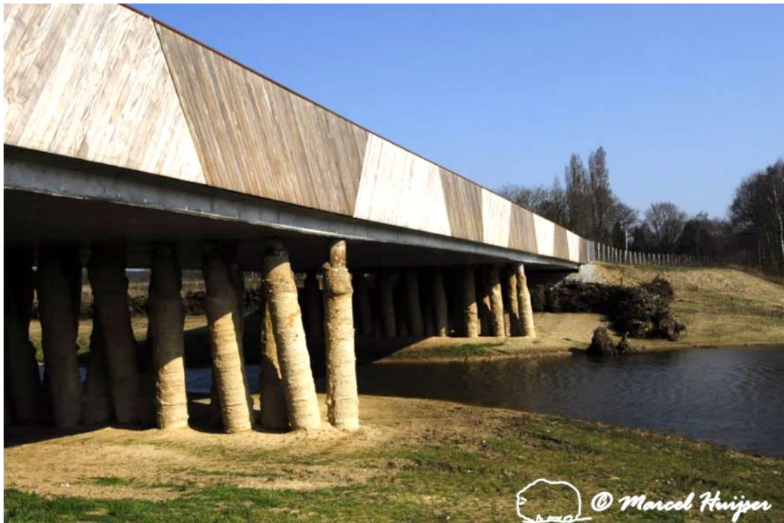
Figure 20. Visual barrier on a multifunctional underpass (water, wildlife), The Netherlands. The fence reduces visual and noise disturbance from traffic for the animals that approach the underpass.
