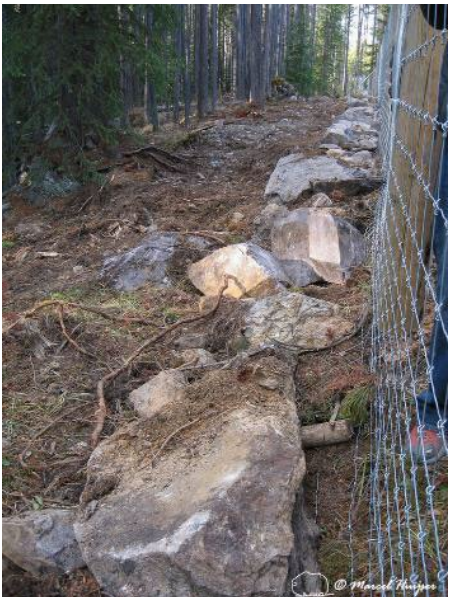
Figure 71. If a dig barrier cannot be dug into the soil, angling it away from the road and covering it with soil and rocks and boulders may be an option. Trans-Canada Highway, Banff National Park, Alberta, Canada.
