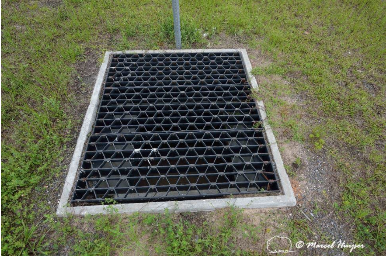
Figure 97. Opening (with bridge grate cover) in median to allow light and moisture in the wildlife underpass Hwy 331 Hwy 83 near Freeport Florida USA.
