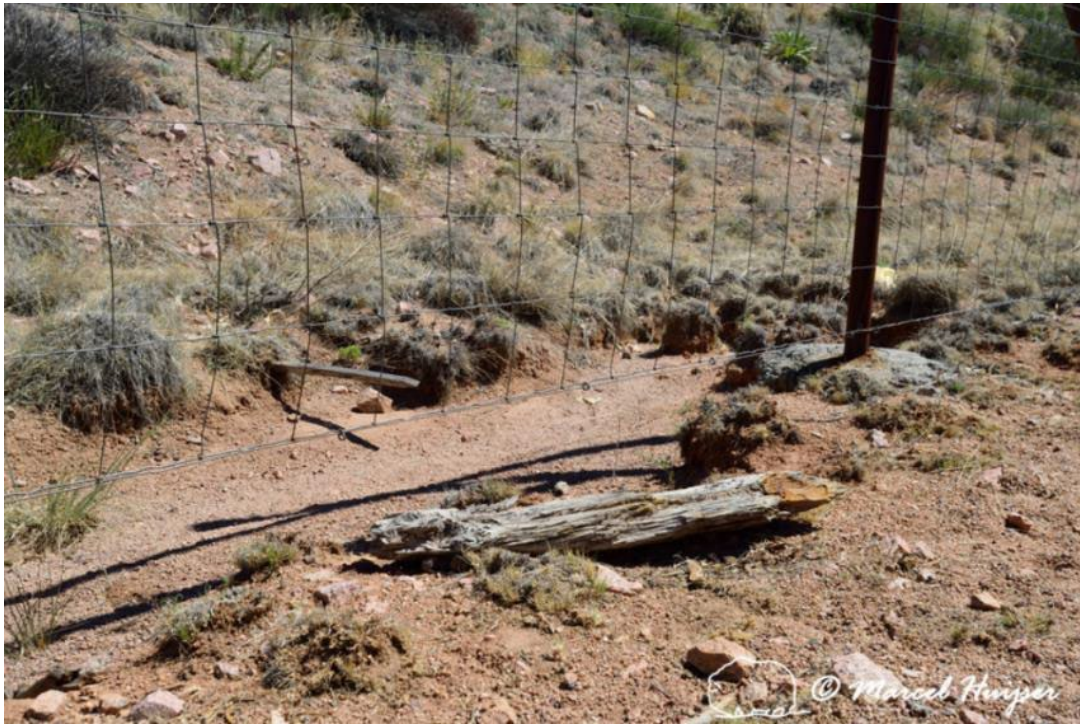
Figure 51. Wildlife fence does not connect to the ground, Arizona, USA. Animals may be able to crawl under the fence.
