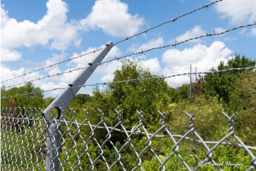
Figure 9. Outrigger on a fence for Florida panther ( Puma concolor coryi ), SR 29, Florida, USA. Note that the outrigger faces the safe side, the habitat side of the fence.
