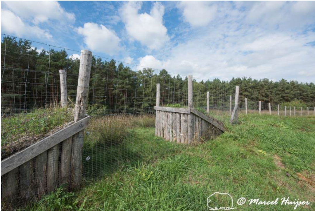
Figure 106. Wildlife fence and jump-out for medium sized mammals and roe deer, along A28 motorway, near Spier, Drenthe, The Netherlands.
