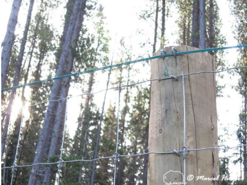
Figure 11. Wildlife fence with high-tensile top wire to reduce damage from falling trees, Trans-Canada Highway, Banff National Park, Alberta, Canada.
