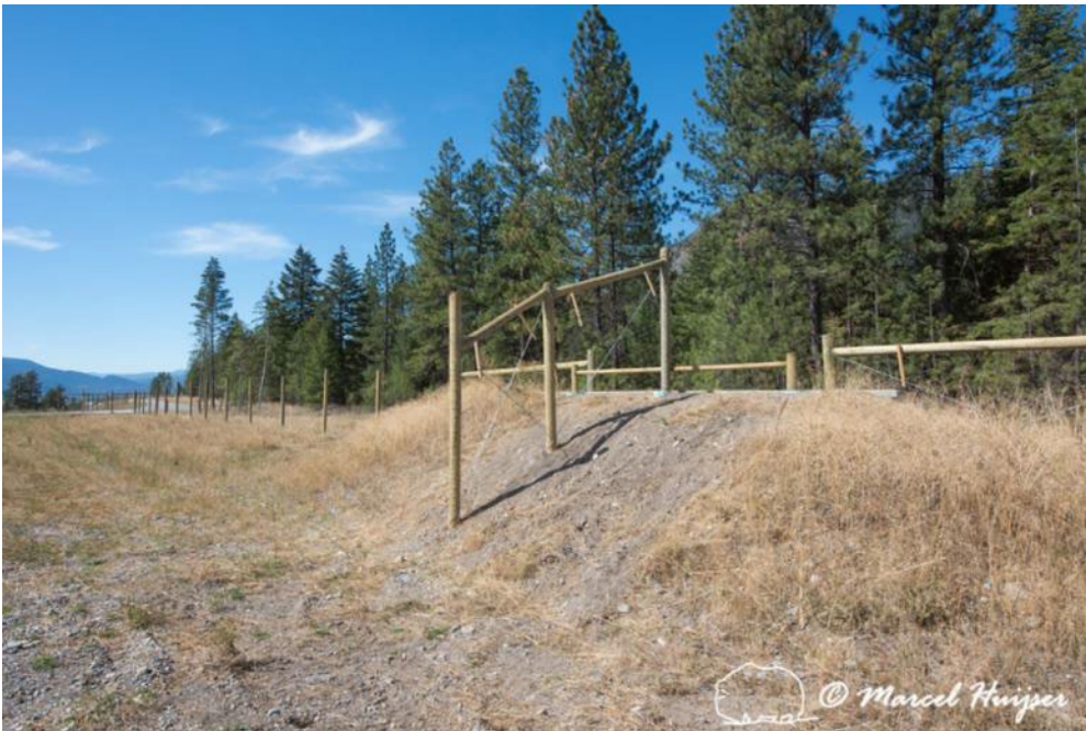
Figure 50. jump-out for bighorn sheep ( Ovis canadensis ) with a short perpendicular fence, near Thompson Falls, Montana, USA. The potential benefits of the perpendicular fence in guiding wildlife to the jump-out are not known.
