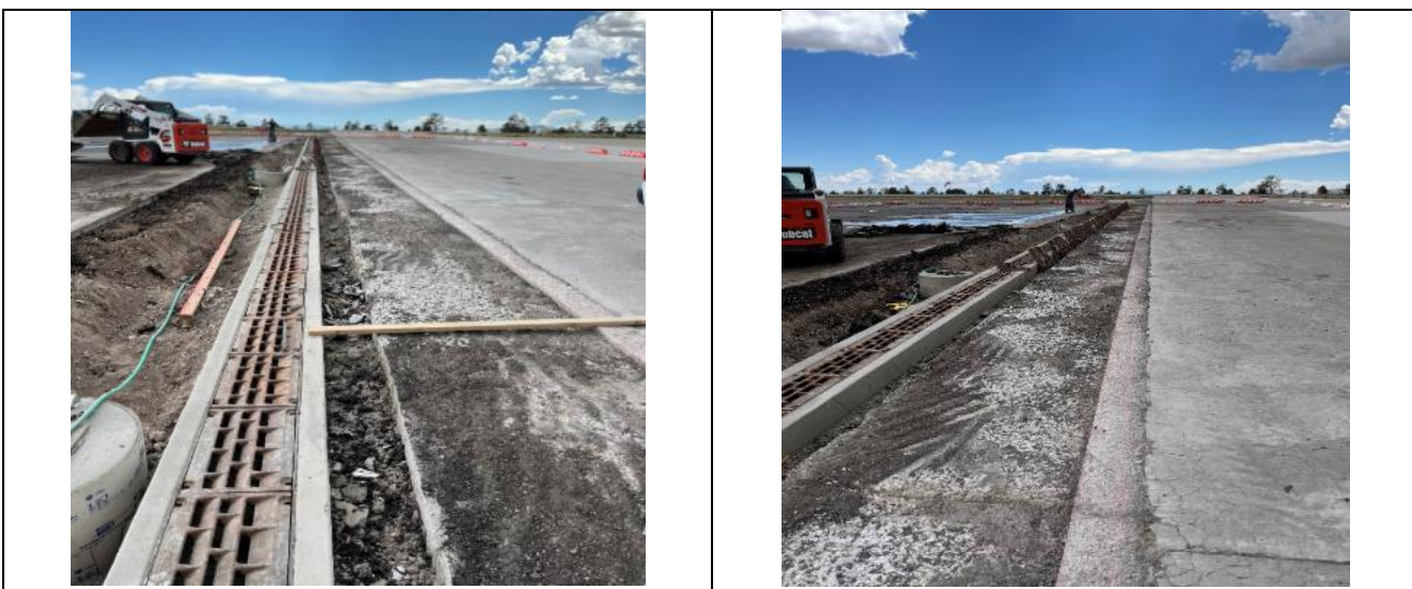
Los Alamos County Airport T-Hangers. Completed trench drain in front of the T-Hangers building footprint.
