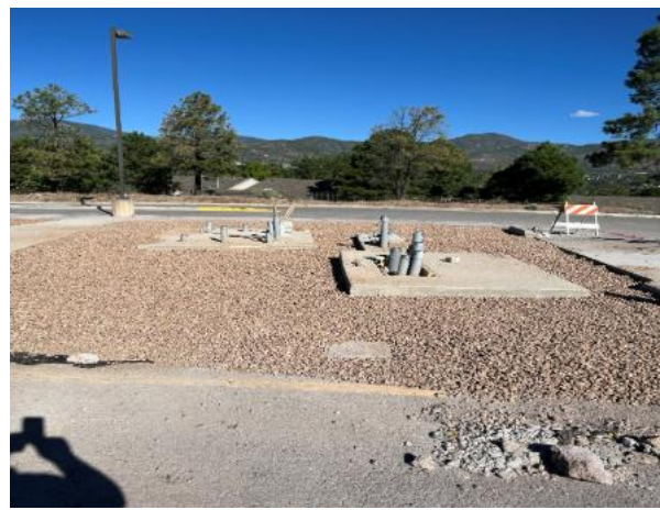
Mesa Public Library EV Chargers. Left panel shows the concrete slab for the accessible charging station. Right panels show concrete pads for the EV charger power blocks.
