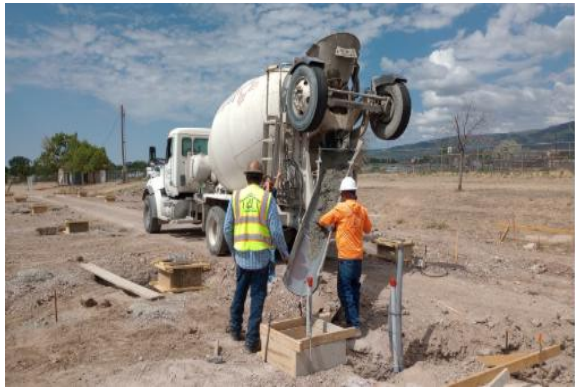
Brewer Arena Improvements. Top panels show the completed restrooms restoration. Left panel shows contractor pouring the piers for the Grandstand and Pavilion
