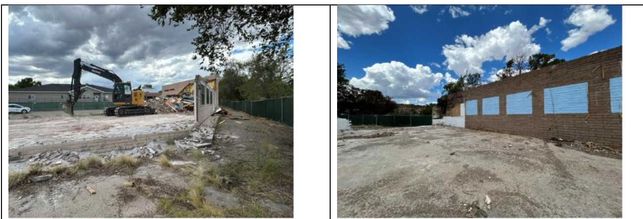
Longview Dr. Buildings Demo. Progress photos showing the footprints of buildings 112 A-C and 124
