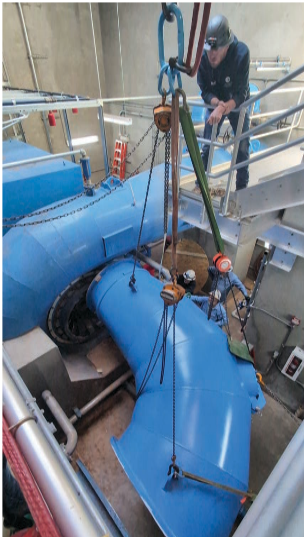
A replacement elbow for the draft tube in Abiquiu’s low flow unit 3 was recently installed.
